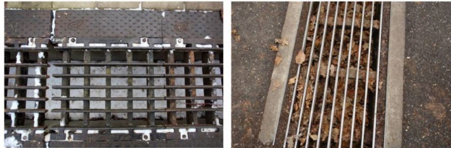
FIGURE 7 | Example of a toad-proof cattle guard ( left ) and one that can still be bridged by toads ( right ). The opening between the road and the first steel bar in the toad-proof cattle guard is 6 vs. 4 cm in the one that can be bridged by toads. Photos: F. Ottburg.
